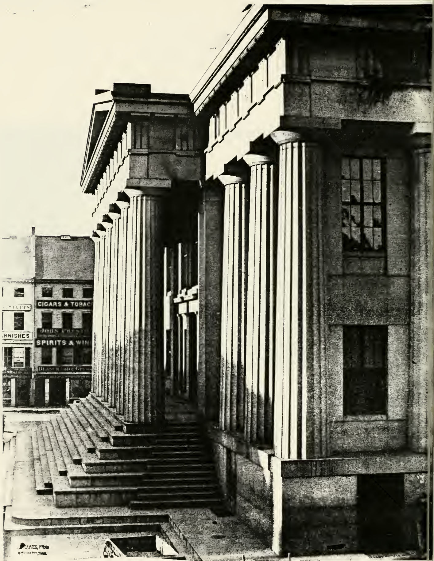
1860* (19) West Portico looking north, showing original arrangement of steps and curb.
